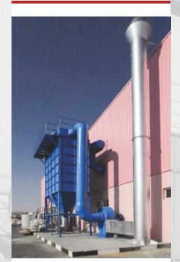
The fumes collected in the fume enclosure are filtered in the bag filter.
