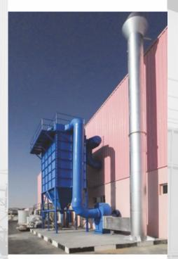
The fumes collected in the fume enclosure are filtered in the bag filter.
