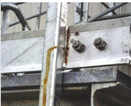
Bleeding and weeping welds
