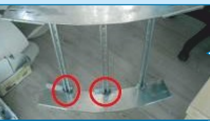
Burned oil during welding
